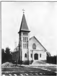
St. Joseph's Roman Catholic Church, Central City, erected 1912
